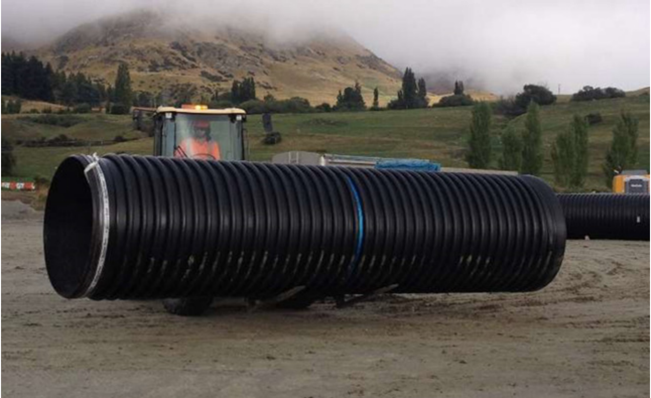
FIG. 5: Pipe has been stropped to the lifting equipment to ensure it cannot be dropped or damaged
